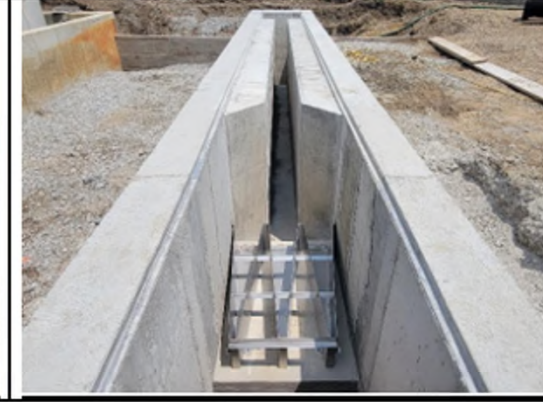
Trapezoidal weir installation – U.V.
