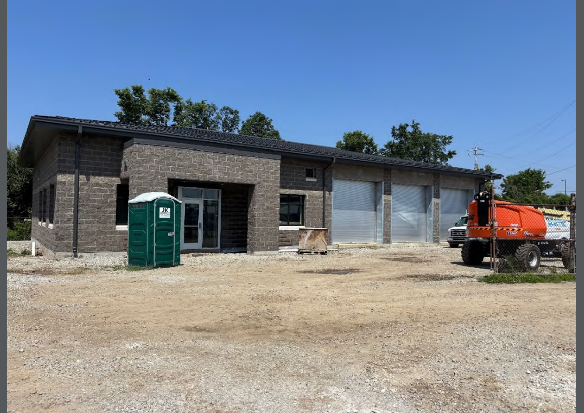
New Admin Building with Garage
