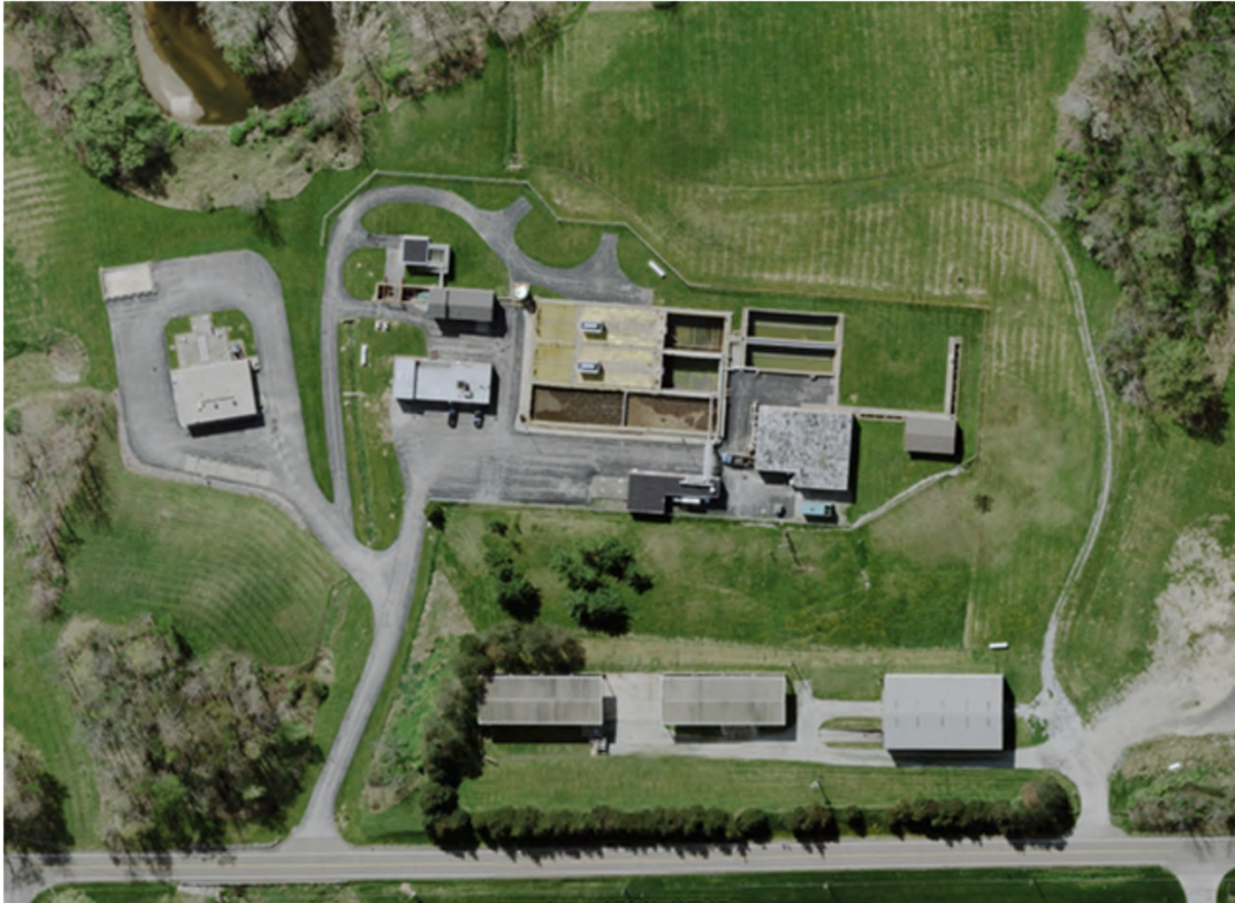
Pre-Construction Aerial View of Existing WWTP
