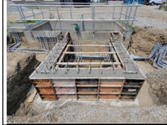
Equipment pad formed wall concrete pour – POST A
