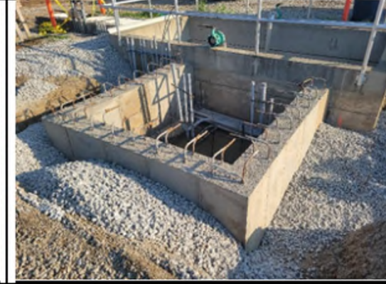
Equipment pad formed walls – POST AERATION
