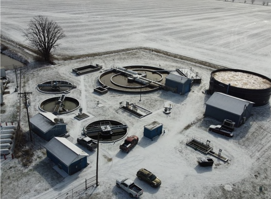
Pre-Construction Aerial View of Existing WWTP
